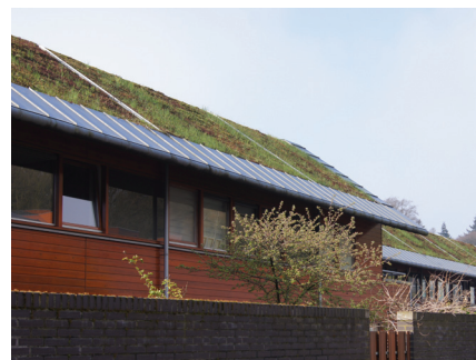
Figur 10: Sedumtag. Monnikenhuizen, Arnhem, Holland. Foto Orbicon.
